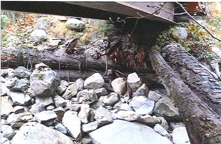
CK2235 Right Abutment 2
