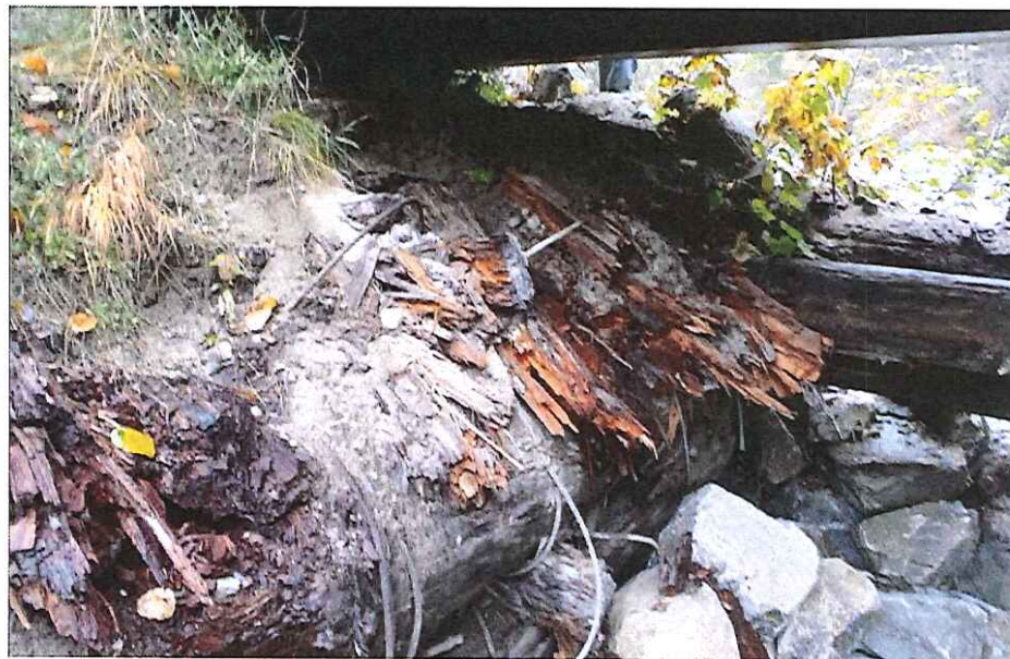
CK2235 Right Abutment 3
