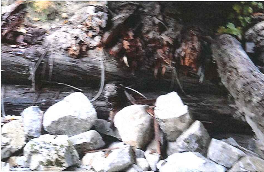
CK2235 Right Abutment
