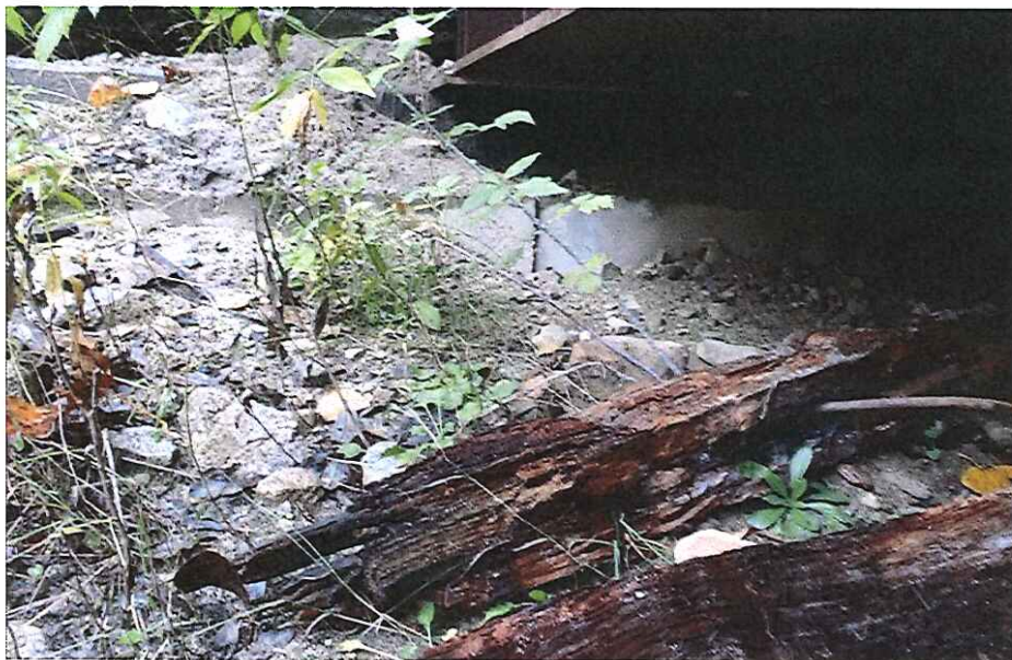
CK2235 Left Abutment
