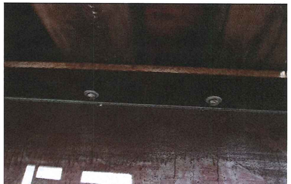
CK2235 Deck to girder bolts
